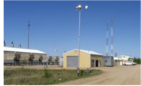
Devon Leismer Compressor Station
